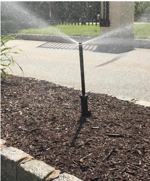
12 inch pop-up spray head - pressurized
