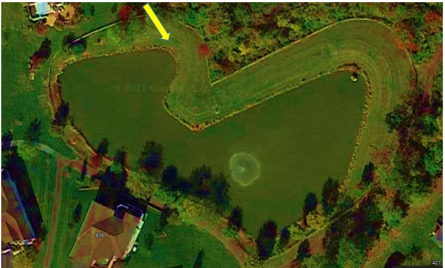
Aerial view of Pond 4 retention basin. Yellow arrow denotes the perspective of the following photo.
