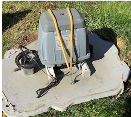
A faux rock enclosure houses the pressurized air source. Unit is a Charles Austen linear diaphragm air pump, model ETX 200, 120 volt, 3.7 amp.
