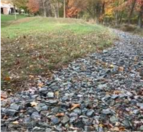
A riprap apron borders the basin's emergency spillway to prevent erosion during severe storms.
