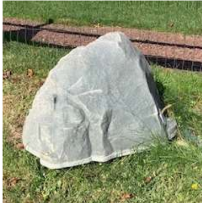
A faux rock enclosure houses the pressurized air source. Unit is a Charles Austen linear diaphragm air pump, model ETX 200, 120 volt, 3.7 amp.
