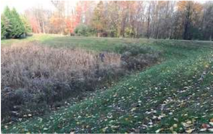
Pond 3 from the perspective of the yellow arrow above. Water-absorbing plantings are thriving in the floor of the basin.
