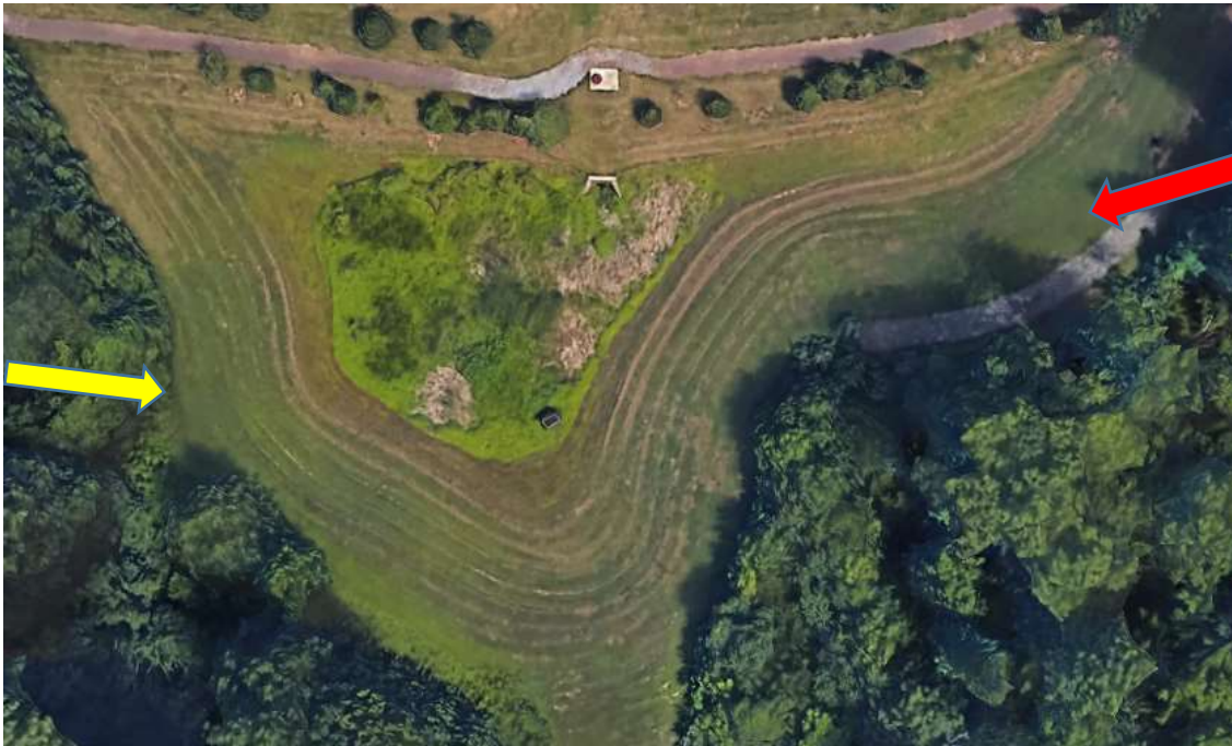
Aerial view of Pond 3 detention basin. Arrows denote the perspective of the following two photos.
