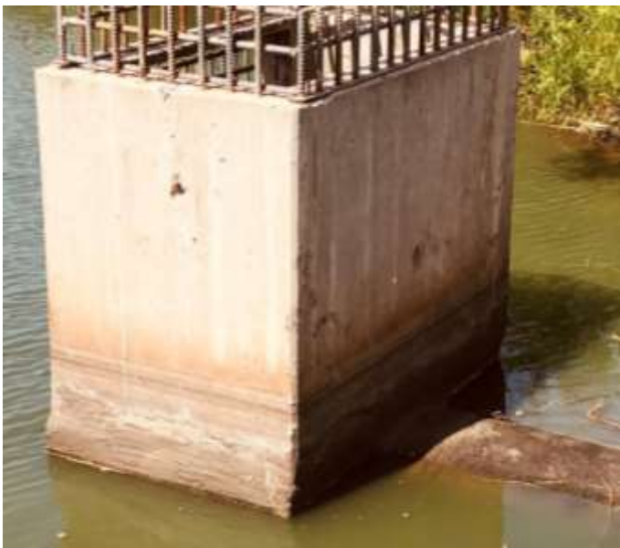
With the repair project complete the pond will gradually refill from precipitation as well as operation of the well pump.
