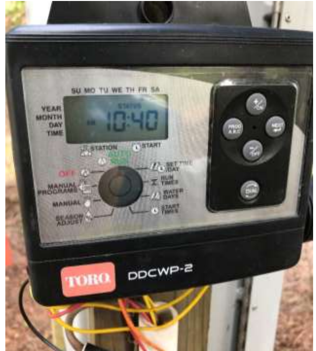
The Toro controller is powered by two 9 volt alkaline batteries and, like the Aquavar unit, remains in place during the winter.
