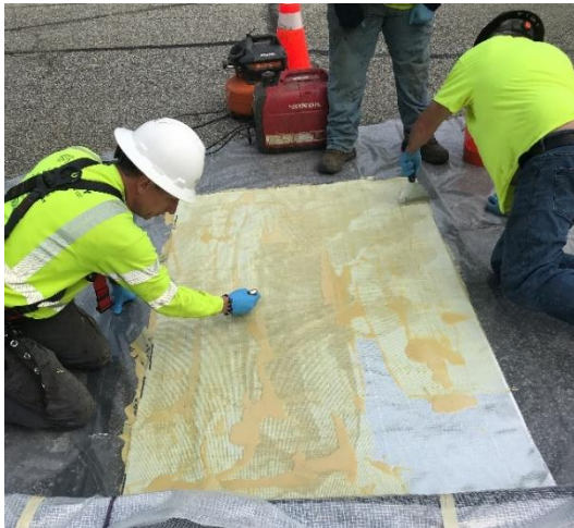
....and then thoroughly spread over both sides of the repair sleeve.
