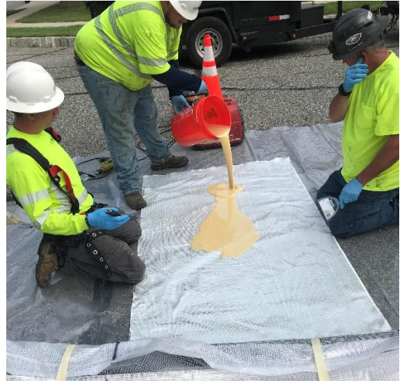
After weighing and mixing the two resin components it is poured onto the sleeve material....
