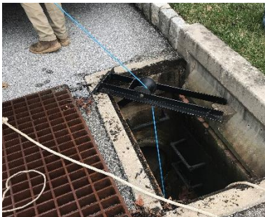
Roller assembly guiding cable
