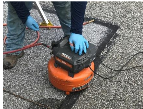
Once in position, the packer is inflated to 30 psi, pressing the sleeve onto the pipe interior wall. A portable compressor (shown) is connected to maintain pressure while the resin cures.
