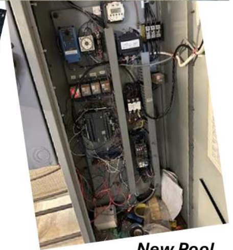
New Pool Control Panel
